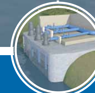
FIRST STAGE PUMPING
