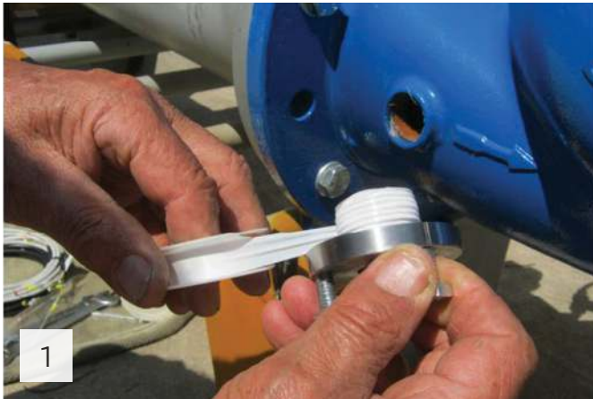
Apply Teflon sealing band on the sealing disk 1" thread
