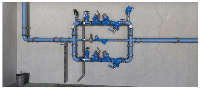
Two-Stage Pressure Reducing Station, featuring BERMAD BC-820-PP-P valves to reduce the incoming pressure by a fixed ratio and share the load with the BERMAD BC-720-P PRV, a redundant, parallel branch to minimize the possibility of total water shut-off and a low flow bypass branch for low demand operation. For information on the other BERMAD products in this system please see the product data sheet for the following components: BERMAD BC-720-P, BERMAD BC-73Q-P and BERMAD BC-80F-P.
