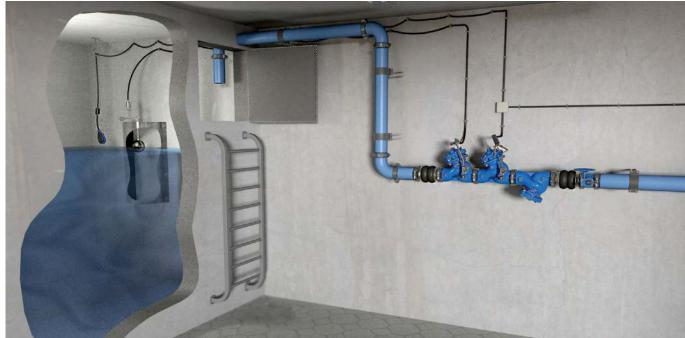
Water Reservoir Level Control System, featuring the BC-750-65-P as an electric controlled backup valve to an hydraulically controlled level control valve.
