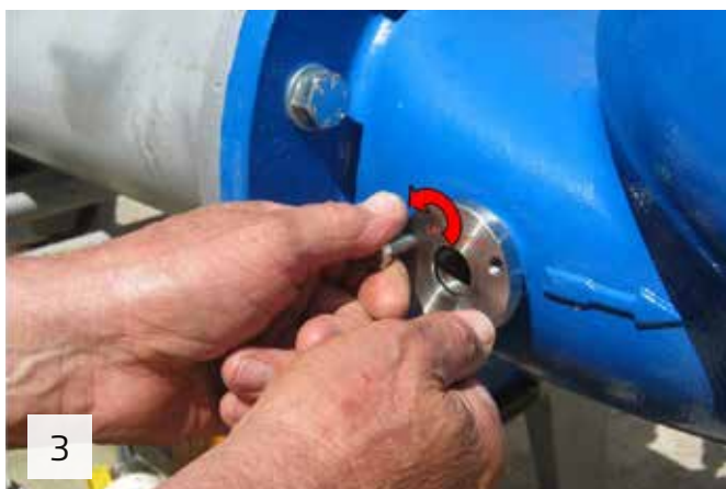
Remove the temporary screws from the disk
