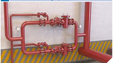
Fire Protection Pressure Reducing system for lower floors in a commercial complex incorporating fail-safe redundancy and pressure relief.
