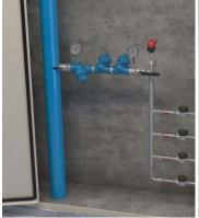
On Floor system supply, secured Pressure Reducing individual direct Pressure System for Potable water.
