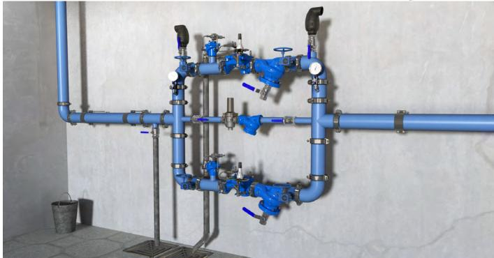
Pressure Reducing Station, featuring BERMAD 43Q valves to relieve excessive downstream pressure, a redundant, parallel branch to minimize the possibility of total water shut-off and a low flow bypass
