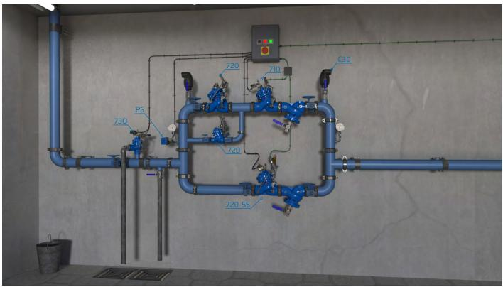
Pressure Reducing Station with Block Valve with Solenoid Control [710] and Automatic Backup PRV [720-55]. In case of abnormal pressure rise detected by the Pressure Switch [PS] the system close
