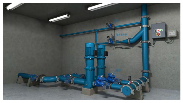
A soft start/stop pump station with emergency surge protection - in a case of power failure the UPS backed controller will activate the 735-55-M to open immediately and anticipate any returning
