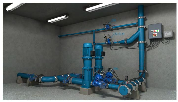
Pump Station, featuring the BERMAD 740 valves to slowly introduce pump pressure to the system or slowly remove pump pressure from the system in response to a signal from the pump controller. In power failure situations, the BERMAD 740 valves will check closed to prevent flow back through the pumps. For information on the other BERMAD products in this system please see the product data sheet for 730 and 735-55.
