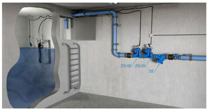
Water Reservoir Level Control System, featuring the 750-65 as an electric controlled backup valve to an hydraulically controlled level control valve. In case of main level control valve malfunction the Electric Float will sense the rise in water level and signal the 750-
