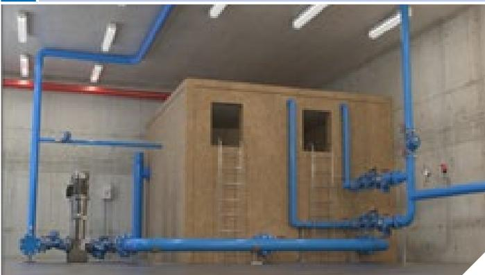
Basement Pump Room, Potable water Reservoir Filling and Level Control System, Pump-Control valves and Active Check valves for Surge prevention, Pressure Relief valve.
