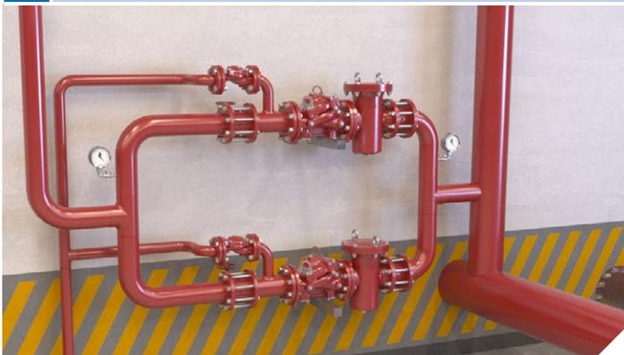
Fire Protection Pressure Reducing system for lower floors in a commercial complex incorporating fail-safe redundancy and pressure relief.
