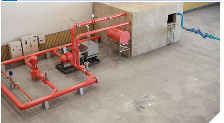
Basement pump room - Reservoir level control with overflow protection, fire protection pumps system with pressure relief valves optional for direct pumping - Suction Control.
