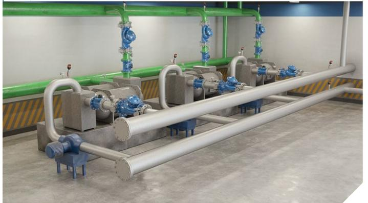
Chillers machine room, individual Chiller Flow & shut off Control, Energy measurement. Balancing between Supply and Return by pressure differential control at end of circulating lines (roof top). Cooling Towers return line flow balance.
