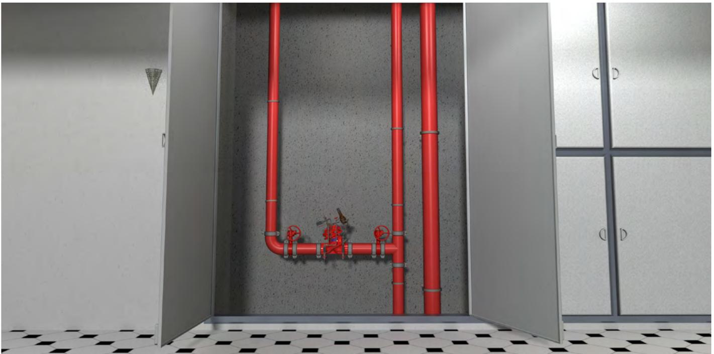
BERMAD BC-791-F0 featured as floor breach containment valve - it will remain fully open under no flow conditions or when supply of fire water to downstream wet pipe system is needed, should downstream pipe line fail, the excessive flow will automatically close the BC-791-F0
