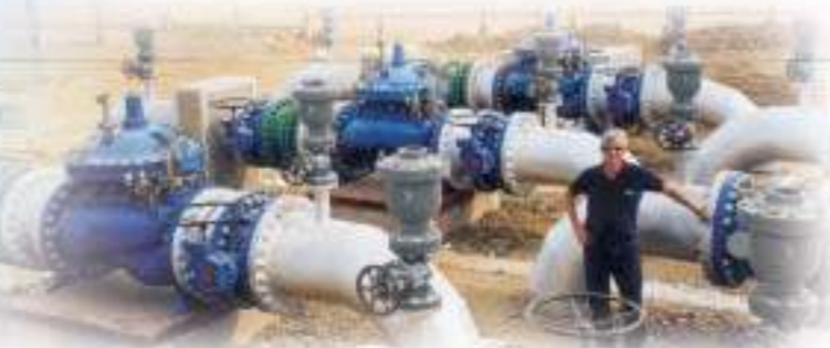
20" industrial reservoir filling system at the entrance to the facility
