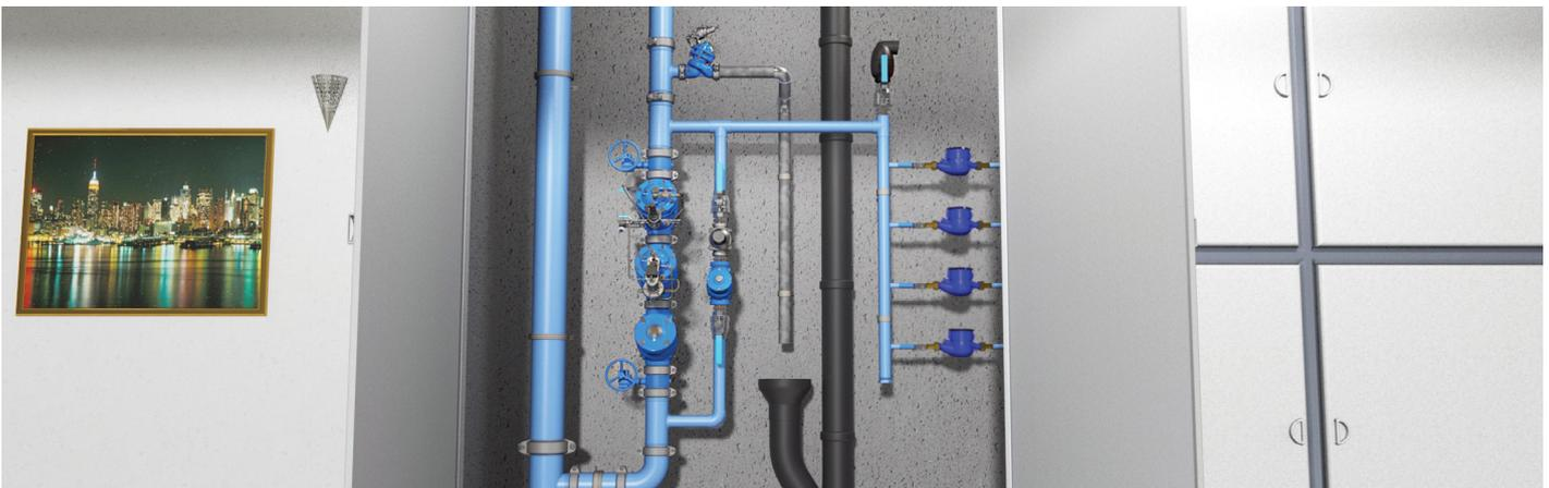
**Pressure Reducing System**, featuring a BERMAD BC-725-H-P system to reduce high incoming pressure to a lower downstream set-point while minimizing the possibility of total water shut-off and a low flow
