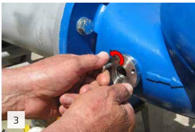
Remove the temporary screws from the disk
