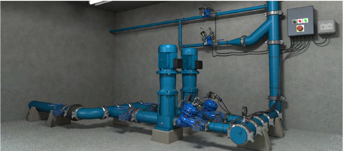
The BERMAD BC-730-P As a pressure sustaining valve that recycles water back to the reservoir at stagnate pump operation, it will remain close when raiser pressure is normal. In an event where the pump works at low flows and high head, the BC-730-P will open to allow sufficient water circulation and pump cooling.
