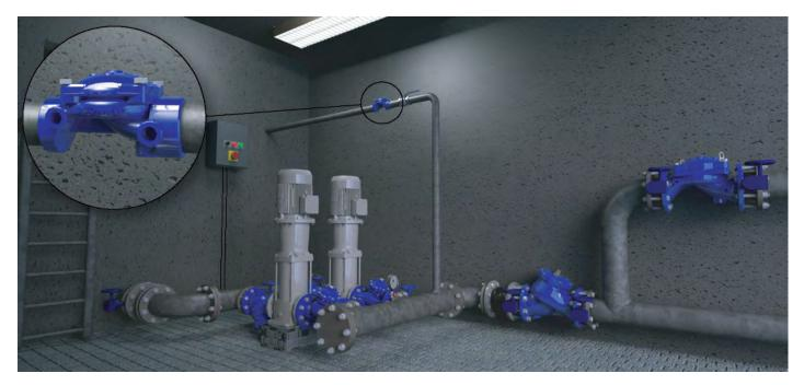
The BERMAD BC-430-P As a pressure sustaining valve that recycles water back to the reservoir at stagnate pump operation, it will remain close when raiser pressure is normal. In an event where the pump works at low flows and high head, the BC-430-P will open to allow
