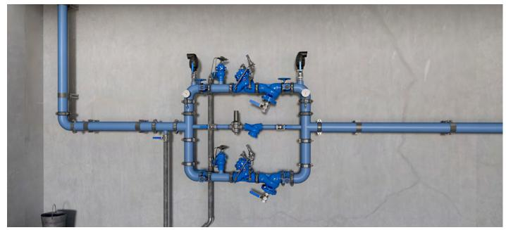
Pressure Reducing Station, featuring BERMAD BC-73Q-P valves to relieve excessive downstream pressure, a redundant, parallel branch to minimize the possibility of total water shut-off and a low flow
