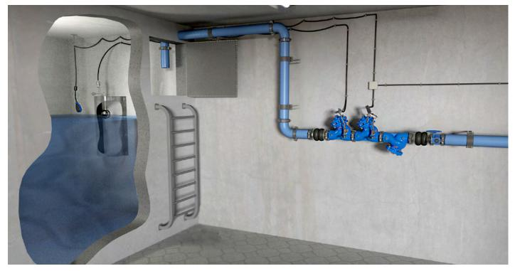
Water Reservoir Level Control System, featuring the BC-750-65-P as an electric controlled backup valve to an hydraulically controlled level control valve. In case of main level control valve malfunction the Electric Float will sense the rise in water level and signal the BC-750-65-P to
