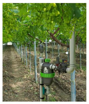
**[1]** BERMAD Model IR-220-50-XZ Opens upon pressure drop, and establishes reduced pressure zone protecting laterals and distribution line.
