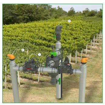
[1] BERMAD Model IR-220-54-X opens upon pressure rise command, and establishes reduced pressure zone protecting laterals and distribution line.
